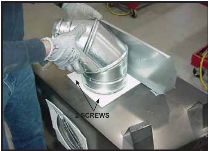
Figure 9.7 To attach the first section of vent pipe, make sure to use the fiberglass gasket to seal between the first vent component and the outer fireplace wrap. Use 2 self tapping screws to secure the gasket to the outer wrap.
